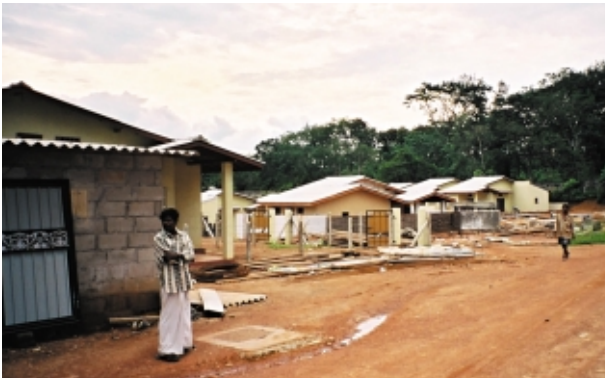
Housing development seen right after the commencement of water supply. (Colombo Southern Towns Water Supply System Extension Project)
